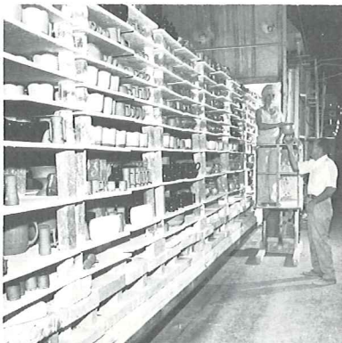
(7) Stacking kiln for firing.
